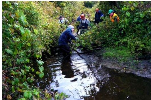
Removing debris restores flow & stops flooding.
