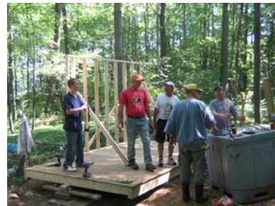
Much rejoicing – a wall is up!
