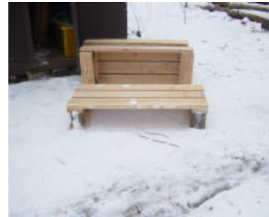
The lunker structure in the foreground sits as it would in the stream; the other in behind shows the “fish-eye” view.
