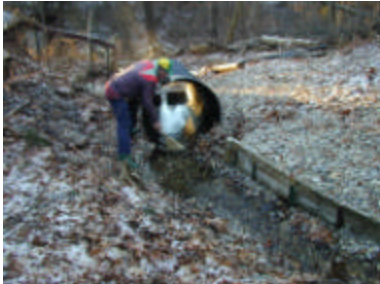
The new spring source is a cleaner set-up allowing easy access for maintenance. Note the increased distance of turbulence to the source pipe for oxygenation.
