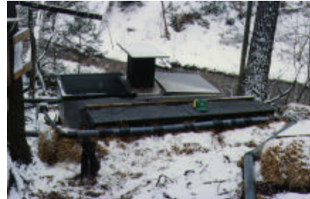
The TRAA has experienced an over 90% success rate with the simple up-welling box pictured above. There are some who say we should go back to this venerable design.
