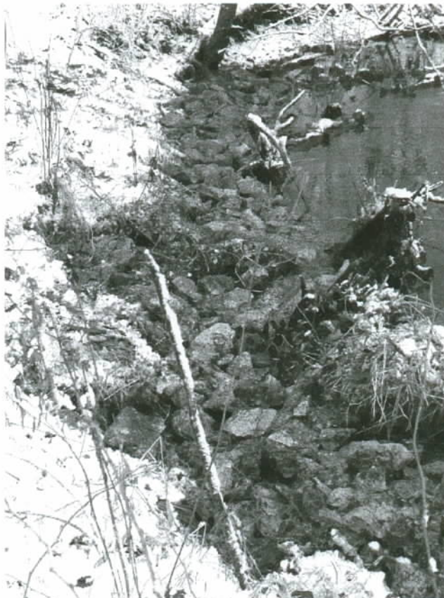
The "cornfield bend" is back-filled - ready for filter cloth, gravel, soil and finally, the planting of vegetation for bank stabilization.
