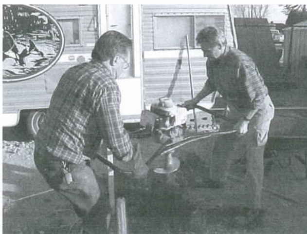
Kevin Lemesurier and Lawson Jones bear down on a post-hole auger for the new fence around the TRAA walleye hatchery compound.
